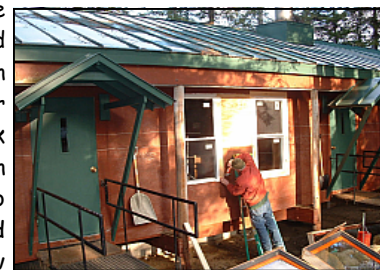
Bob Collins working on the windows
