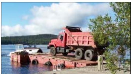
Barge delivering stone
